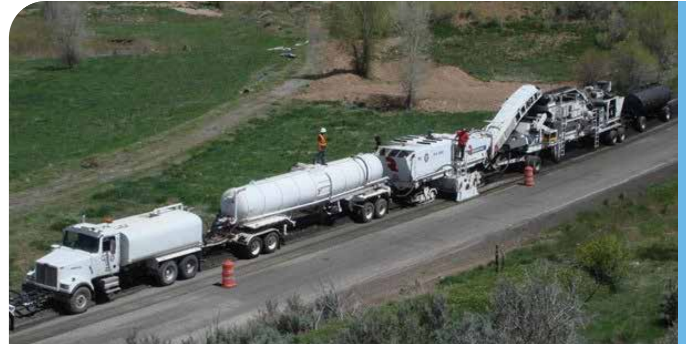
Figure 16 – Cold In Place Recycling, partial depth, multi-unit train
