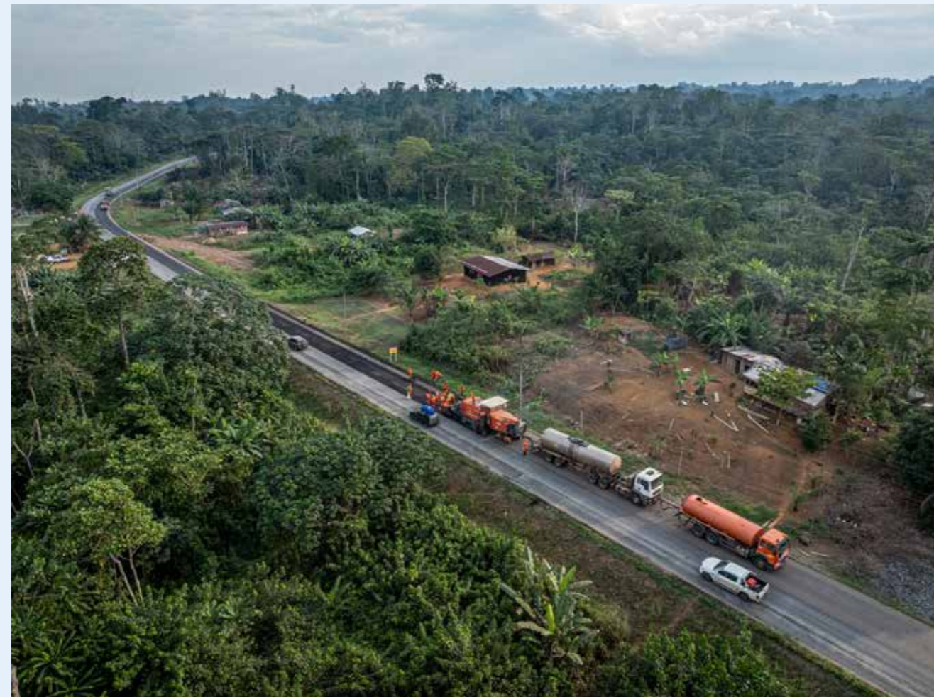
Figure 32 - Cold in-place recycling of pavement with bitumen emulsion
