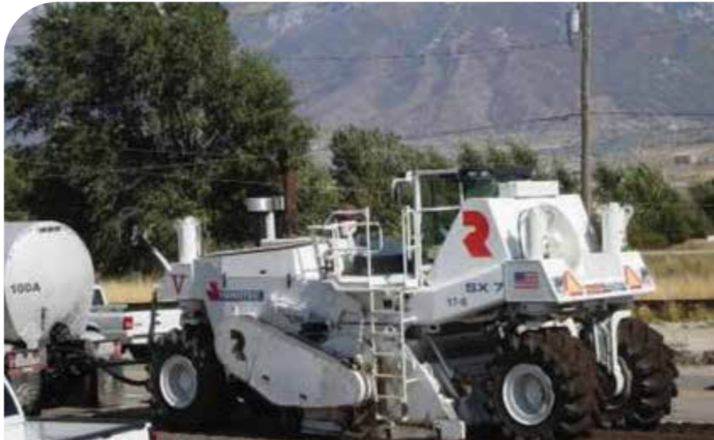
Top: Figure 17 – CCPR plant Bottom: Figure 18 – Full depth reclamation
