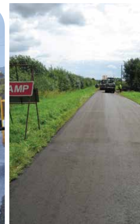
Figure 29 - CCPR final surface
