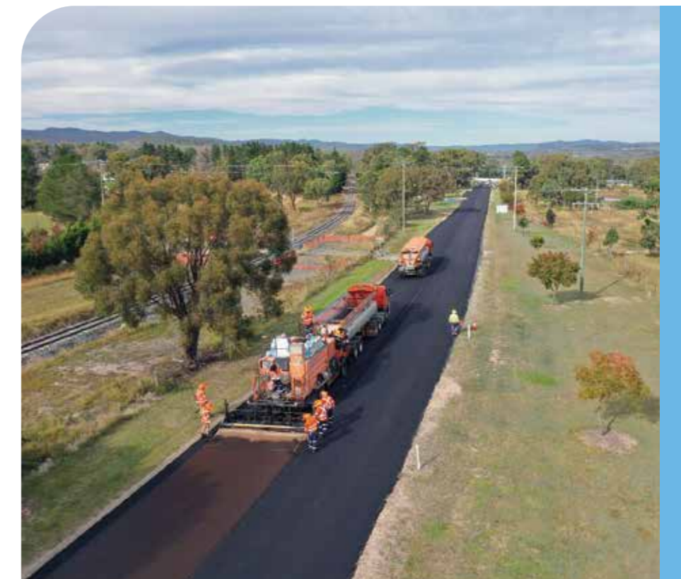
Figure 9 - Application of microsurfacing
