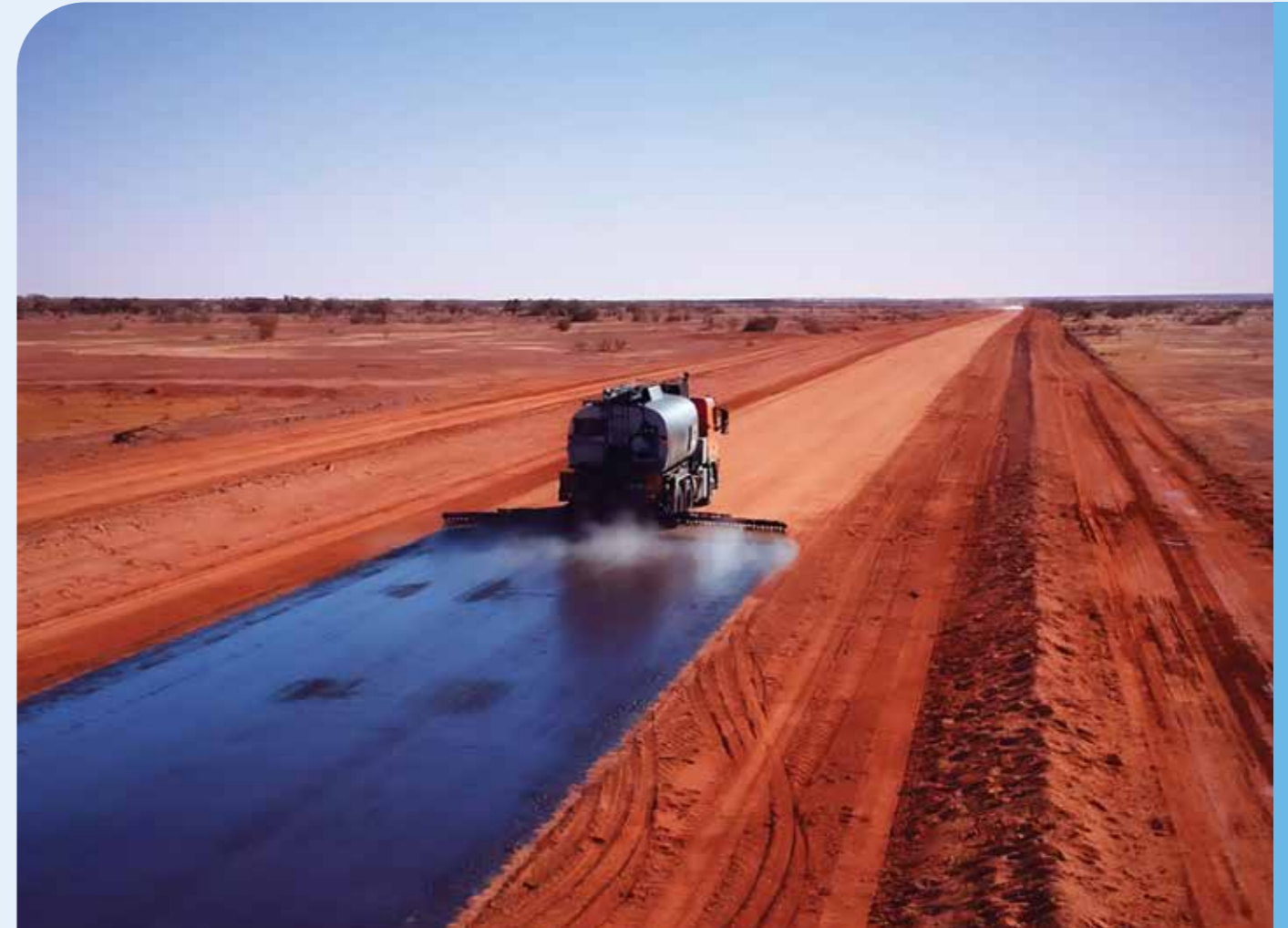
Figure 1 – Application of prime coat
