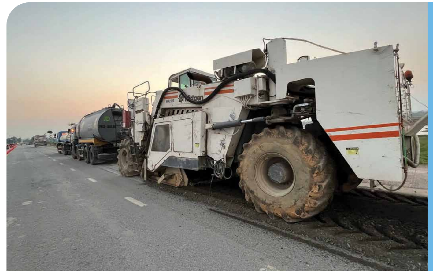
Figure 23 - Cold in place recycling, Vietnam
