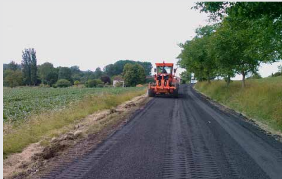
Figure 10 - Application of gravel emulsion
