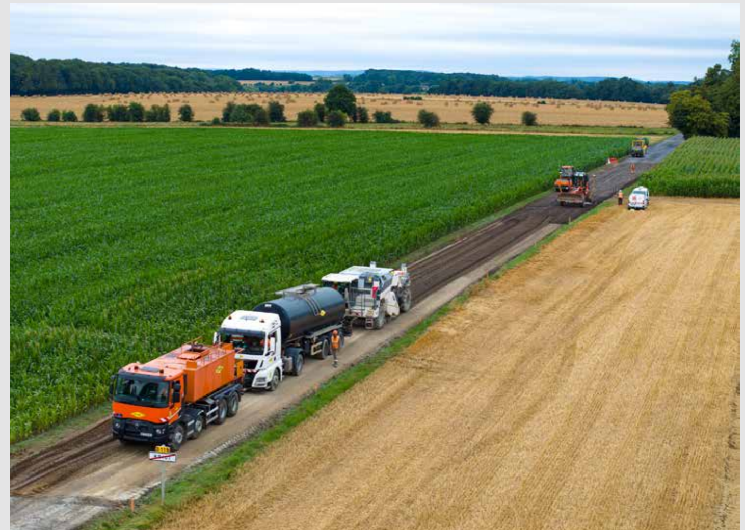
Figure 30 – Road stabilisation with bitumen emulsion
