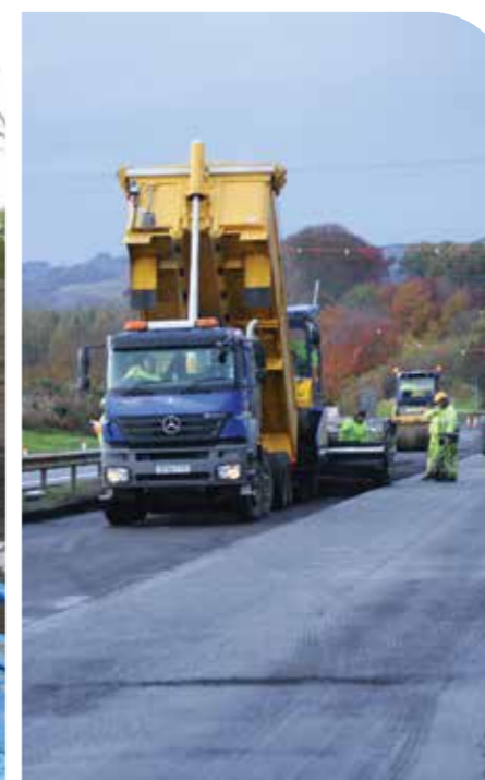
Figure 28 - CCPR installation
