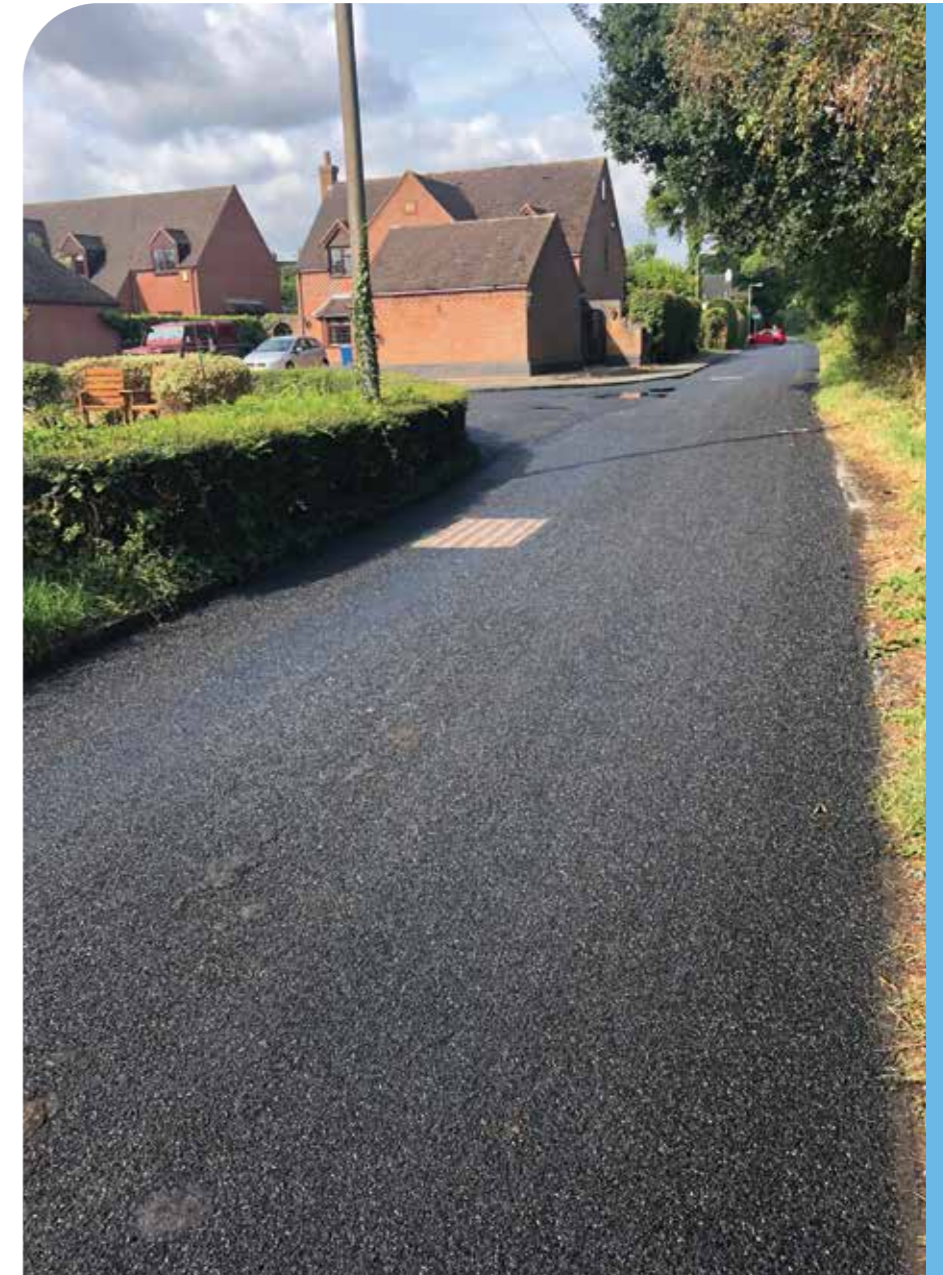
Figure 5 - Fog seal on surface dressing in rural setting
