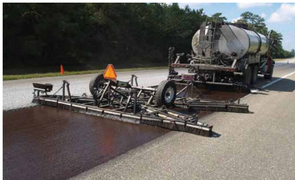
Top: Figure 6 - Application of chipping in surface dressing Bottom: Figure 7 - Scrub seal overview
