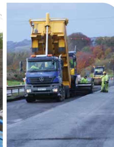
Figure 28 - Pose du CCPR
