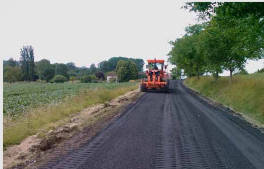
Figure 10 - Application de grave émulsion
