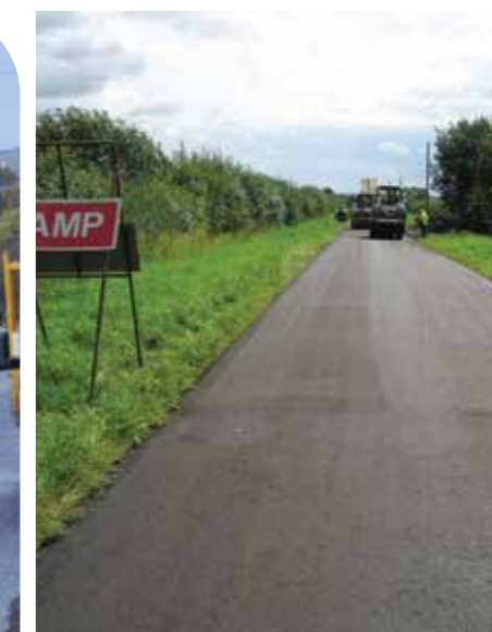
Figure 29 - Surface finale du CCPR
