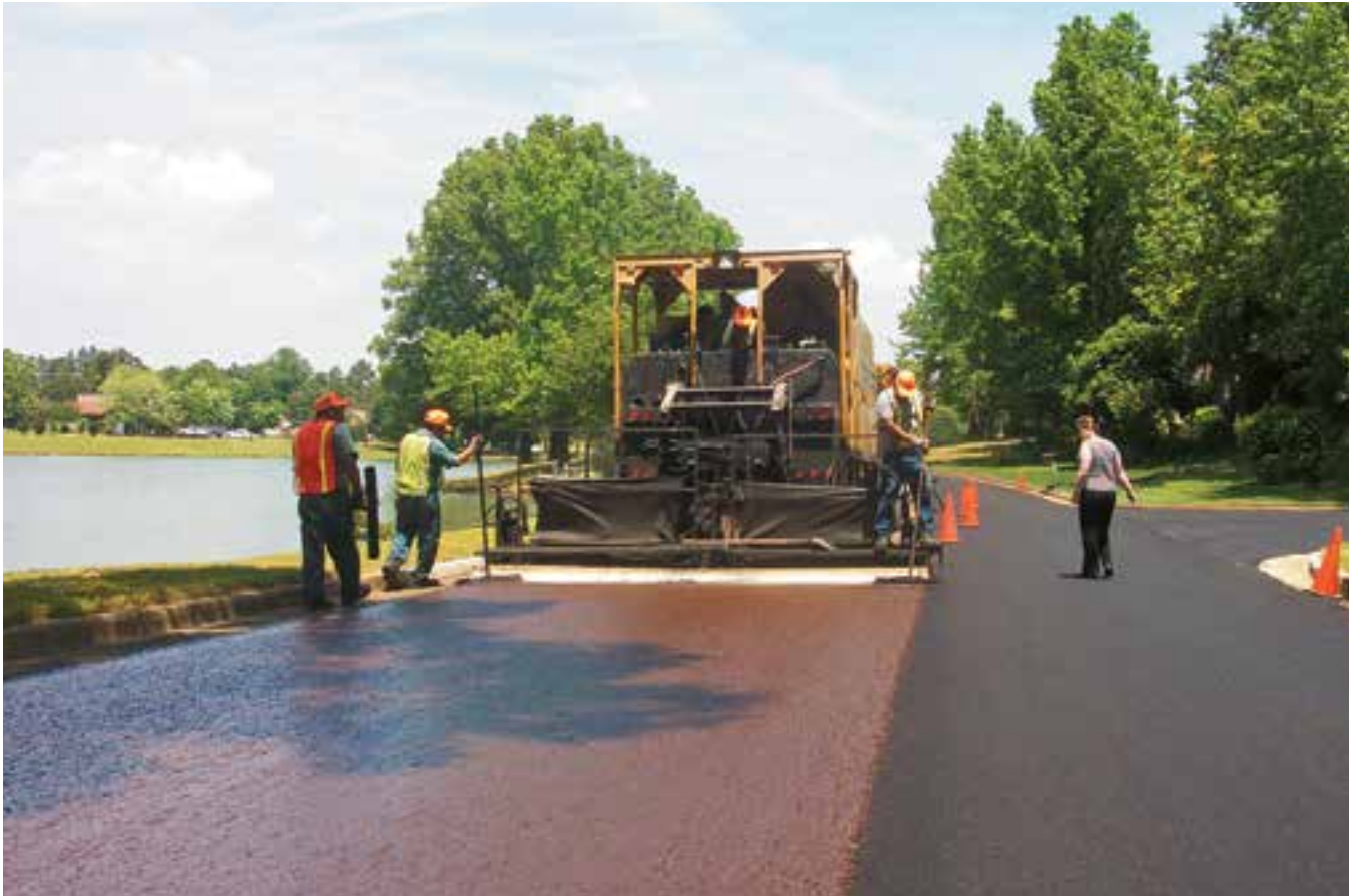
Asphalt emulsion containing polymer modifier is integral part of micro surfacing placed on suburban street
