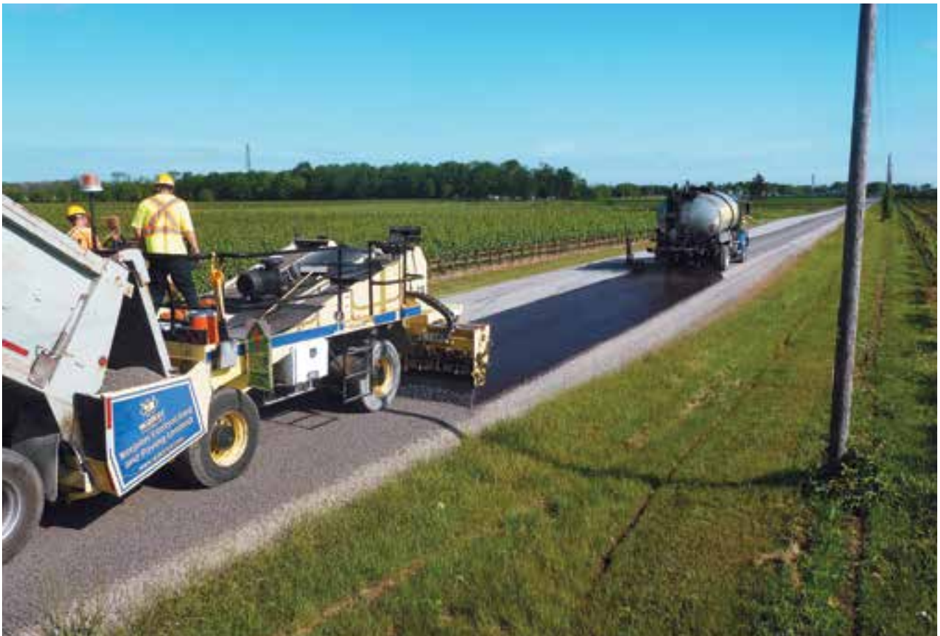
Rural chip seal: chips are placed uniformly across asphalt emulsion placed by distributor truck
