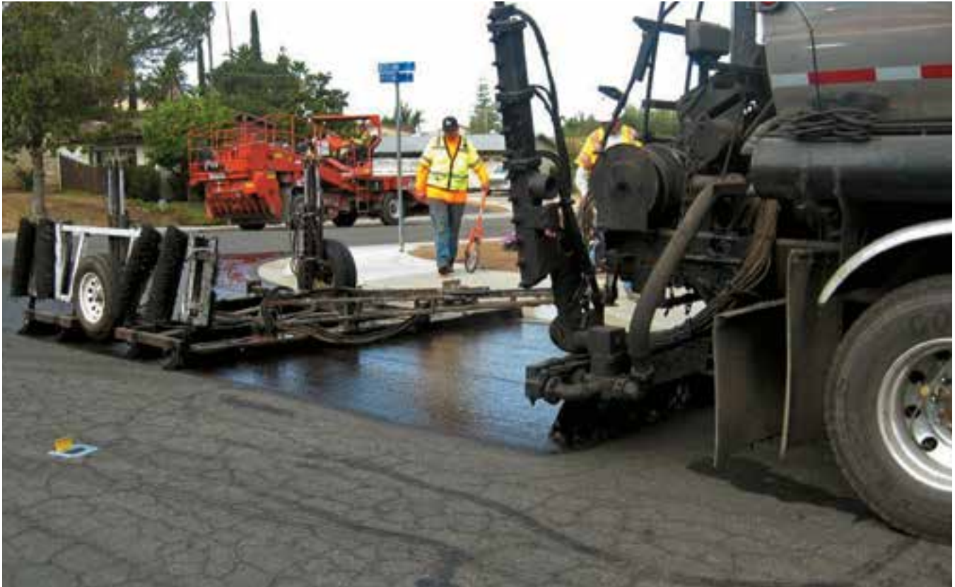
For Escondido, Calif., scrub seal, polymer modified emulsion is placed in advance of trailer with brushes that will work emulsion into pavement; chips will follow
