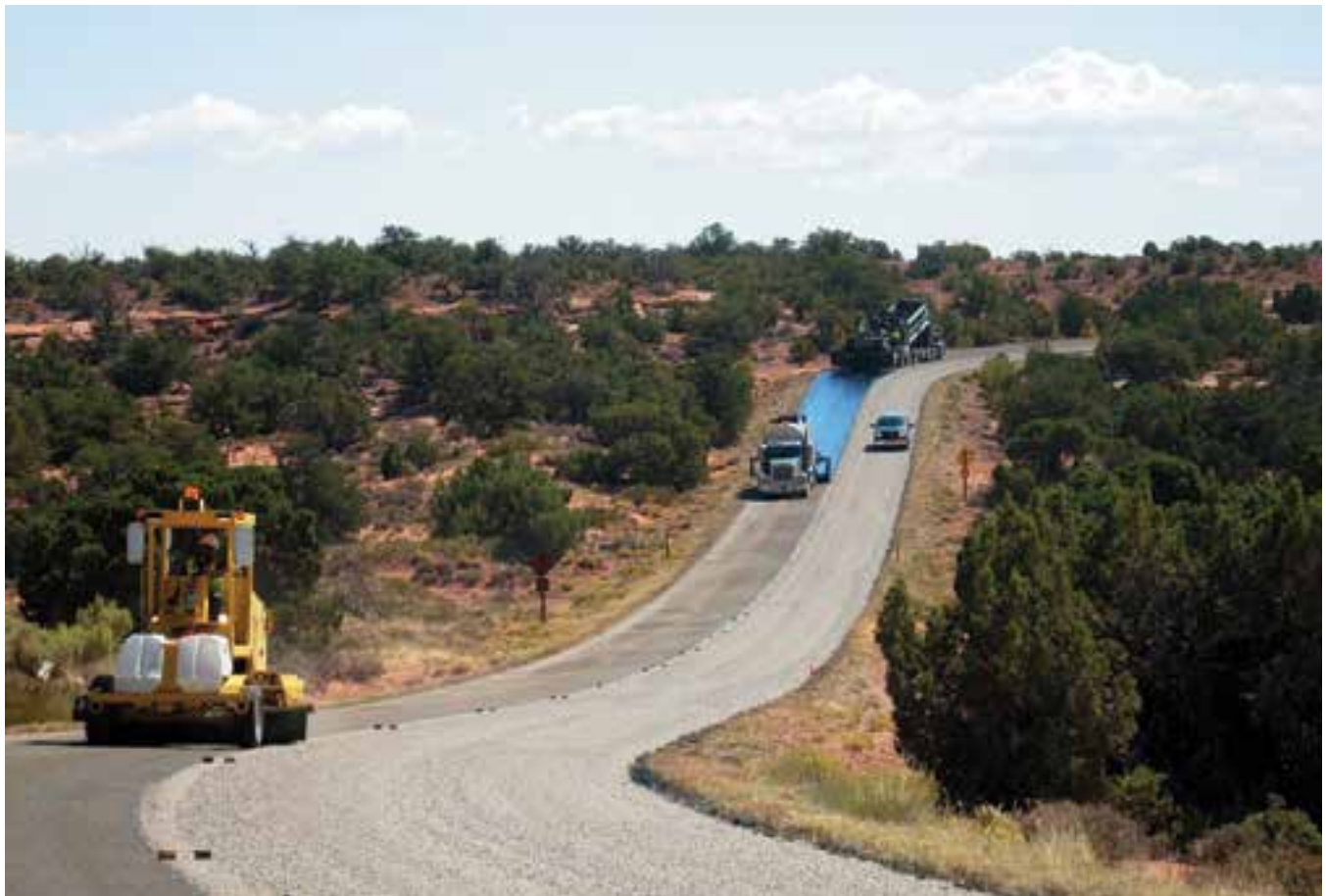
Canyonlands National Park was among four scenic Utah parks to receive polymer modified asphalt emulsion chip seals
