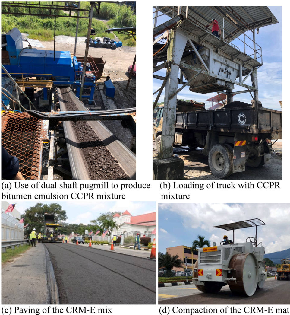
Fig. 5. Production and placement of the bitumen emulsion CCPR mixture.
