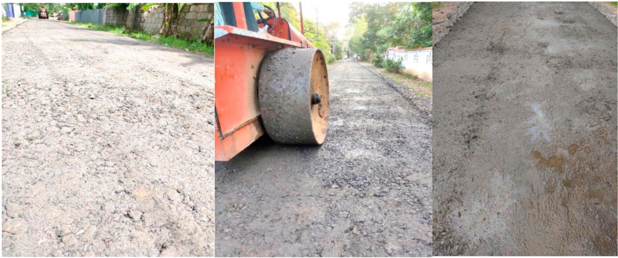
Figure 3. Section S2, S3 and S4 – ETB mixes with virgin aggregates.
