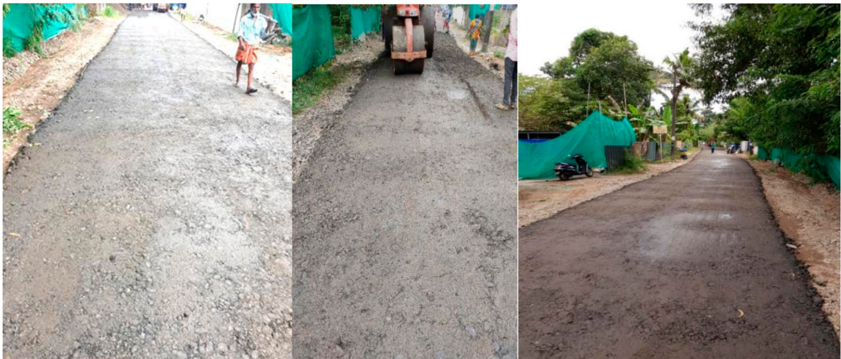
Figure 4. Section S5, S6 and S7 – ETB mixes incorporating 50% RAP.
