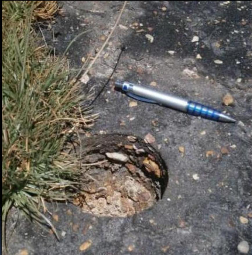
Pavement condition before rehabilitación. Original sand/asphalt built in 1978. 10 to 15 cm thick.
