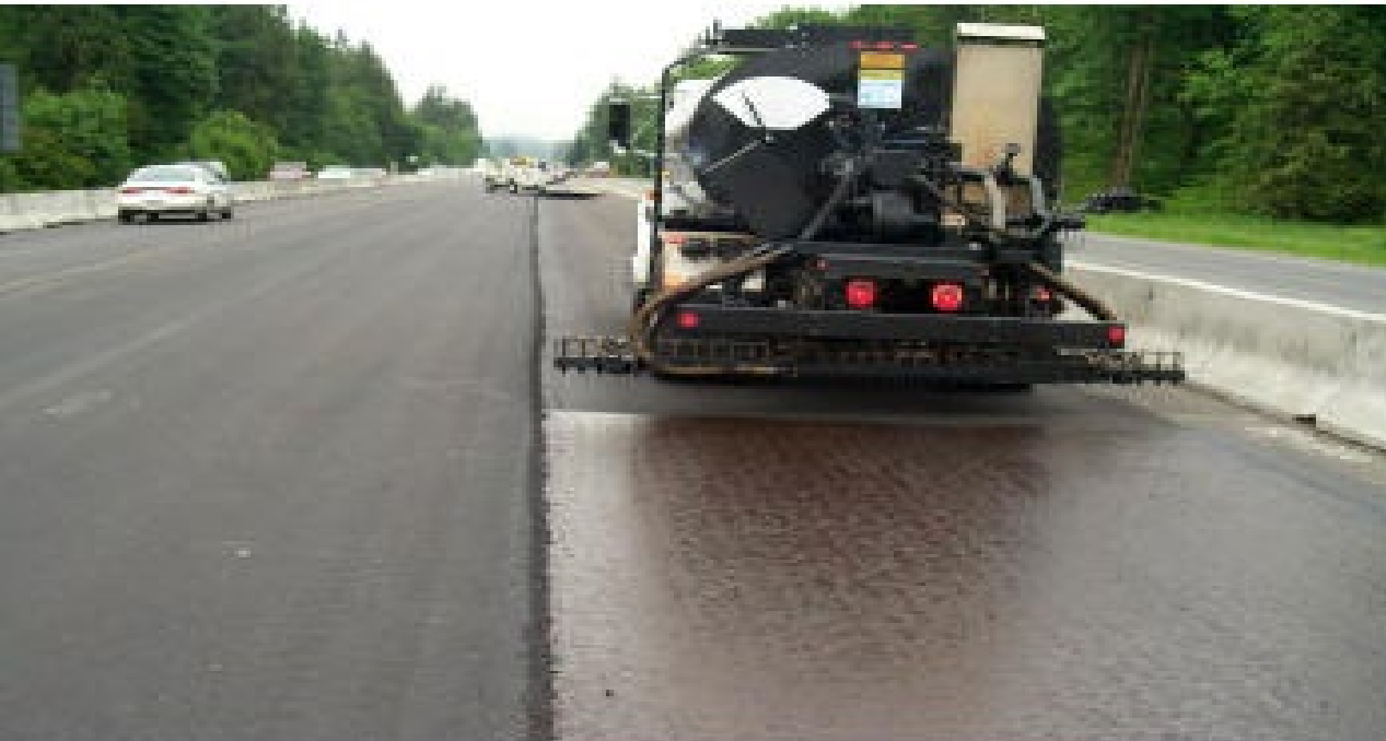
Figure 1. Good tack coat coverage.
