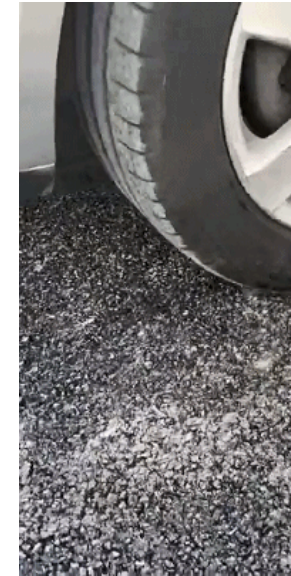
Short curing period after. compaction
